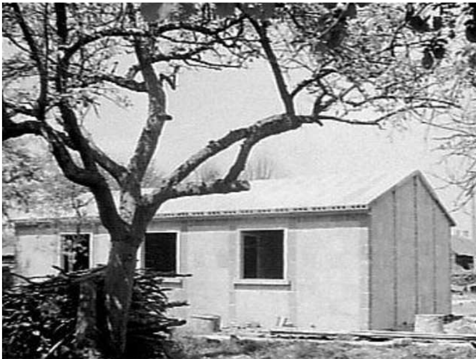
Afb: Maycrete woning in Eindhoven
